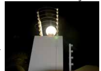
Example of bad installation of outdoor street lighting
