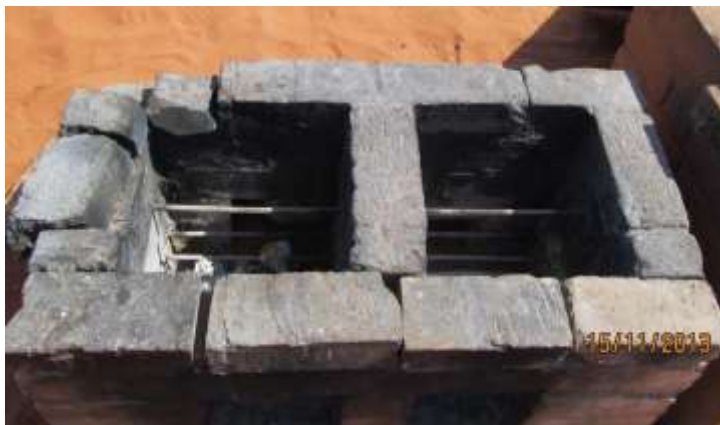
Photo 5. NaDEET's demonstration energy efficient fireplace
