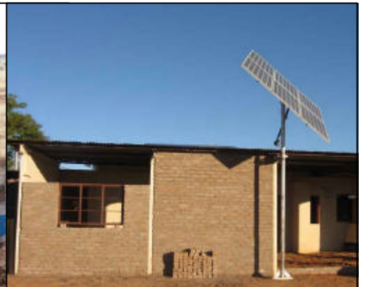
The new communal living area
