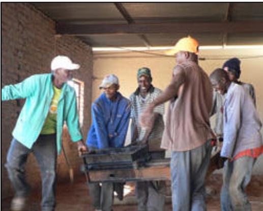
Builders moving the generator frame
