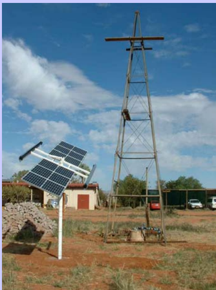
Solar water pump at NaDEET's base
